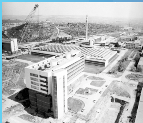
Construction of Pavilion Z, Bohunice premises, 80s of the 20th century
